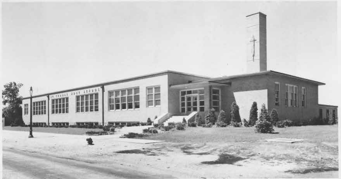
Original School Building. Notice the single floor - of course, more students meant more school.
